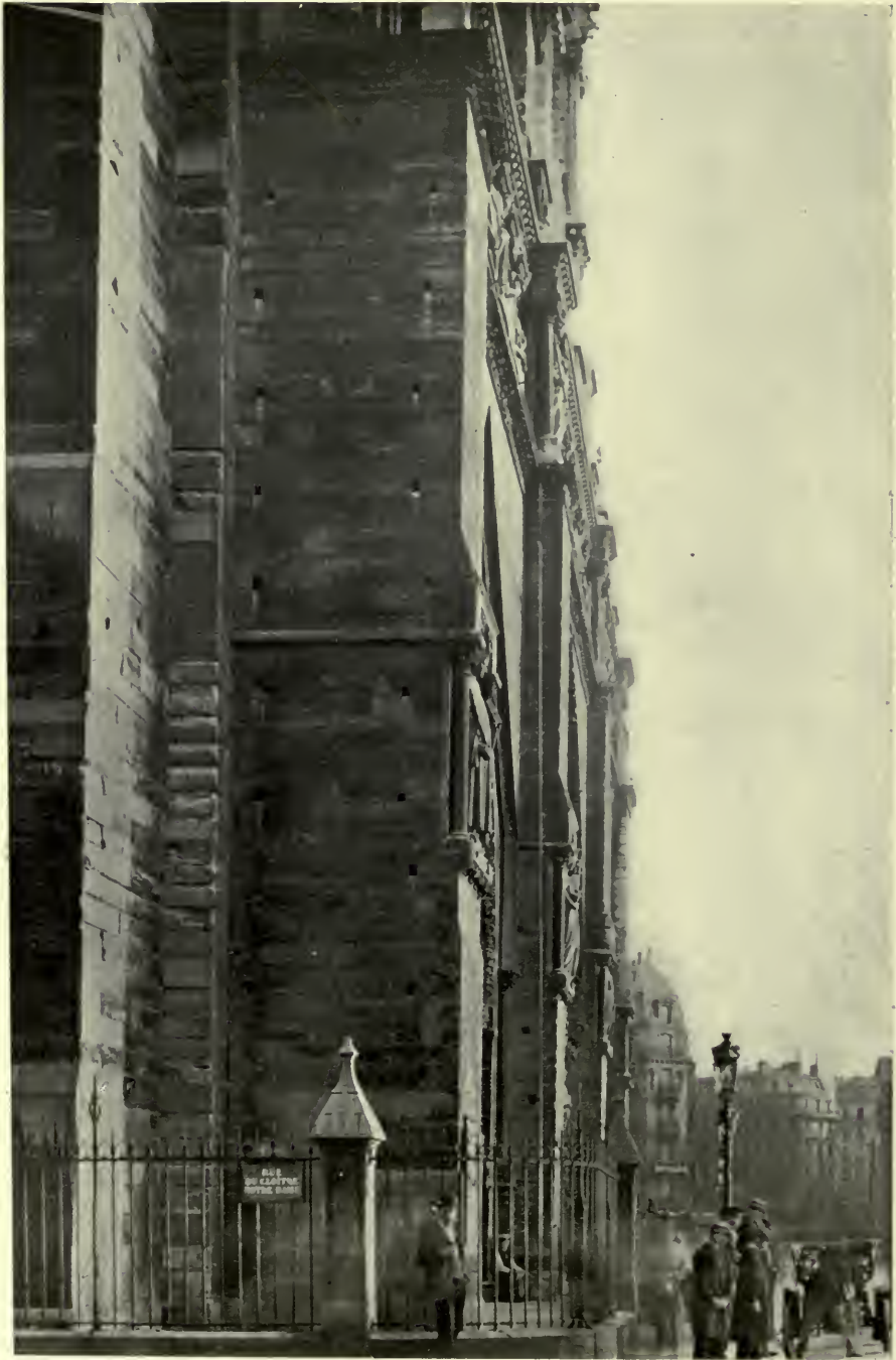
FIG. 5. THE LEANING LOWER FAÇADE OF NOTRE-DAME.
